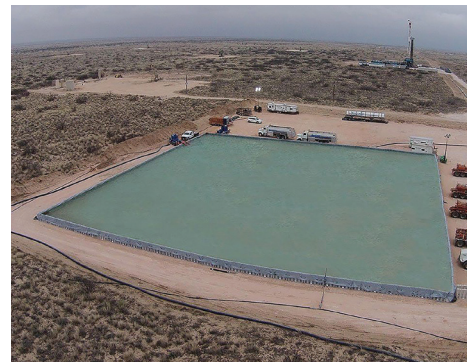
Primary & Secondary Containment
