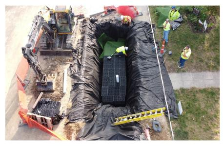
Steve Krehbiel, Quick Supply and our engineer, Bill Murphy, assisted with the installation of a FocalPoint high-performance modular biofiltration system for this project.
