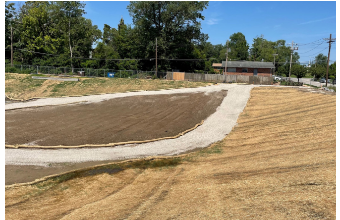
Flexamat infilled with aggregate for the site access roads.
