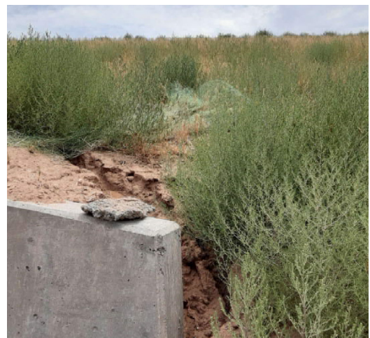
Plastic netting that has grown up with the tumble weeds, causing the washout behind the box wingwall.
