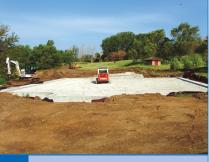
Geotextile and aggregate bedding installed.
