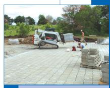
PaveDrain can be driven on immediately.
