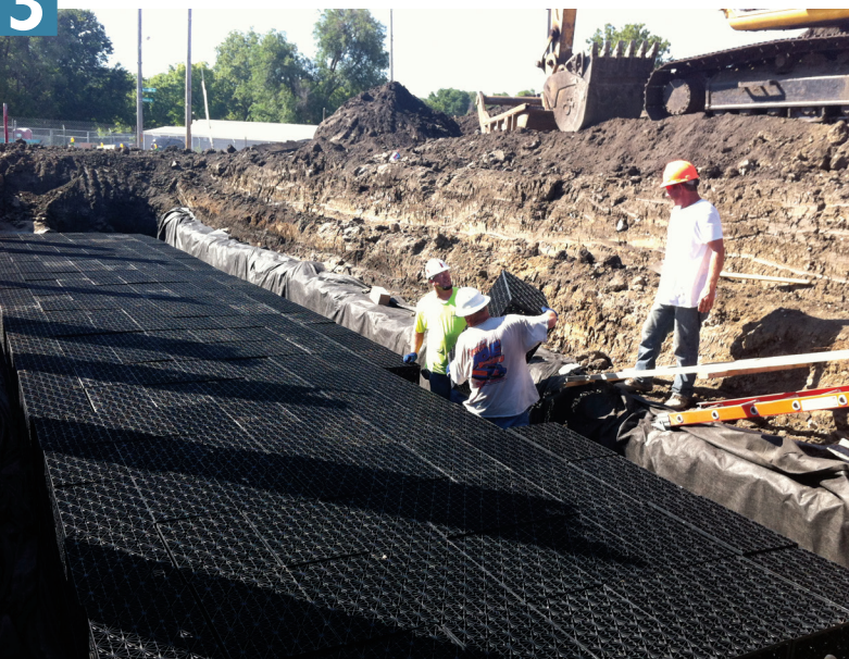
3 The lightweight modular tanks are easy to maneuver and install.
