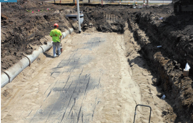
7 Sides are backfilled & compacted to 95% proctor.
