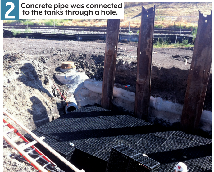
3 The lightweight modular tanks are easy to maneuver and install.
