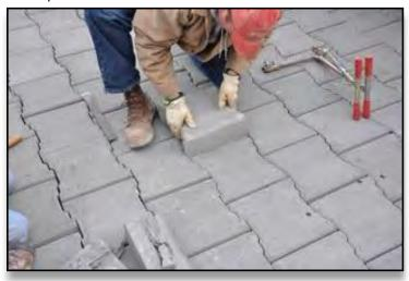
Slide the new block down into place. You may use a rubber mallet to tamp it down securely at the edges, be sure not to damage the new block by using your 3 lbs. hammer!
