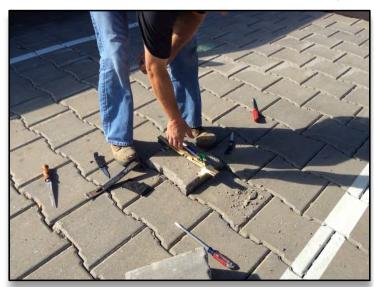
Once the damaged block is removed, debris should be cleaned out of area. Use the PaveDrain extractor to install the new block.
