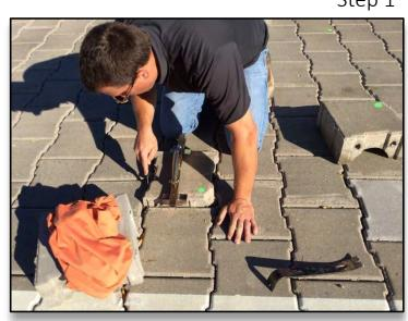
\*\*The Polyester cables (as shown in Step 1 above) can be cut and removed. It will not affect the performance of the PaveDrain system.
