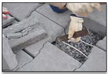
Break out the block using a 3 lbs. hammer, being careful not to damage any of the adjacent blocks. It is best to start in the middle of the block and work your way out. A concrete masonry chisel can help as well.
