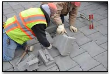
Now that the damaged block is fully removed, you are ready to install the new block. Line up the replacement block to fit the hole where the old block was.
