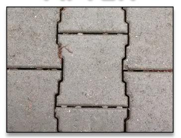
Just one pass of an Elgin Whirlwind Vacuum Truck over the PaveDrain System filled with mulch and road debris.
