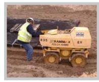
Fig. 23 Vibratory compaction of side backfill is ALWAYS REQUIRED, regardless of what backfill material is used.
