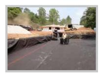
Fig. 7 Use a string line and marking paint to square the system footprint.
