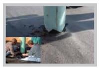
19 Cut an "X" into textile to accomodate pipe penetration and seal with a boot.
