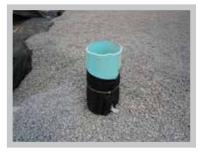
Fig. 17 Install port into R-Tank®.
