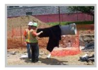
Fig. 22 Seal the pipe boot with the included band clamps and duct tape.
