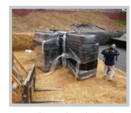
Fig. 3 Installation can be sped up by either assembling the tanks in the excavation or placing the pre-assembled tanks in the excavation.
