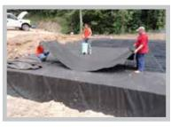
Fig. 20 Encapsulate R-Tanks® with geotextile.
