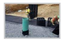
Fig. 11 Installed Inspection Port
