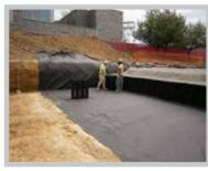
Fig. 5 Pull wrinkles out of geotextiles so material lays flat.
