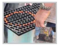
Fig. 12 Cut the horizontal plates to accommodate all ports.
