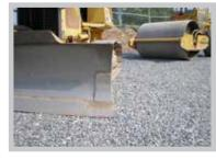
Fig. 4 Base must be smooth to ensure units fit together without gaps.
