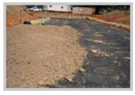
Fig. 26 Pushing backfill parallel to the Geogrid prevents the grid from shoving.
