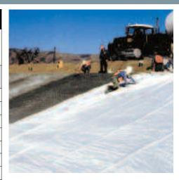
Hydrotex Linings, Mats, and Armor Units are filled in place by pumping fine aggregate concrete into fabric forms. The results are reduced material and equipment costs, faster installation, and dependable erosion and scour prevention.
