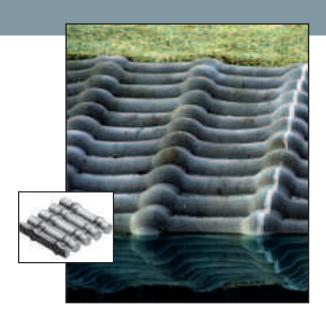
rap, gabions, precast concrete blocks, and conventional concrete slope paving because of several factors. It can mitigate uplift forces due to outflow and excess pore water pressure, reduce hydraulic uplift by slowing channel velocities, and conform to soil contours to reduce the potential for scour.
