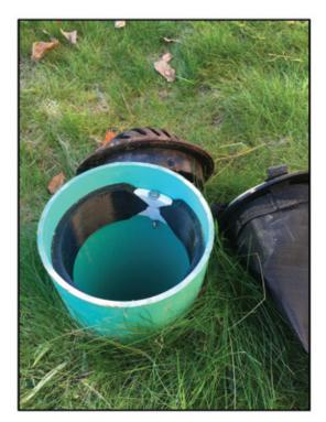
Beehive Filters all have a bypass/over flow built in as shown above.
