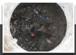
Easy Access Clean out using vacuum truck -access through manholes or hatches at the top of the structure
