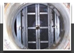
**Upper screen Lids** prevent loss of debris during high flow rain events
