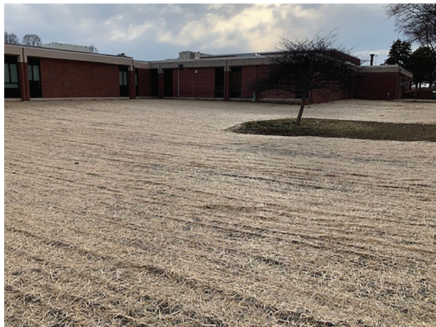
43 Blankets in 8 Hours with Staple Wasp vs. 12 Blankets in 8 Hours with Conventional Installation
