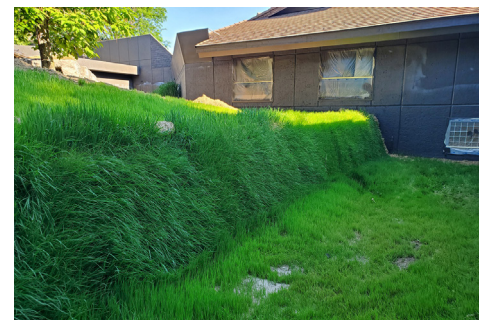
Flex MSE Wall at Henry Doorly Zoo's Gorilla Exhibit - Supplied by ASP Enterprises
