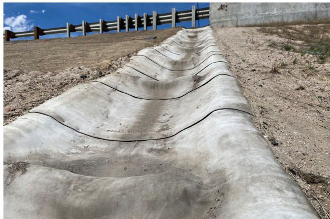
Concrete Canvas® Laid Transversely Across the Channel
