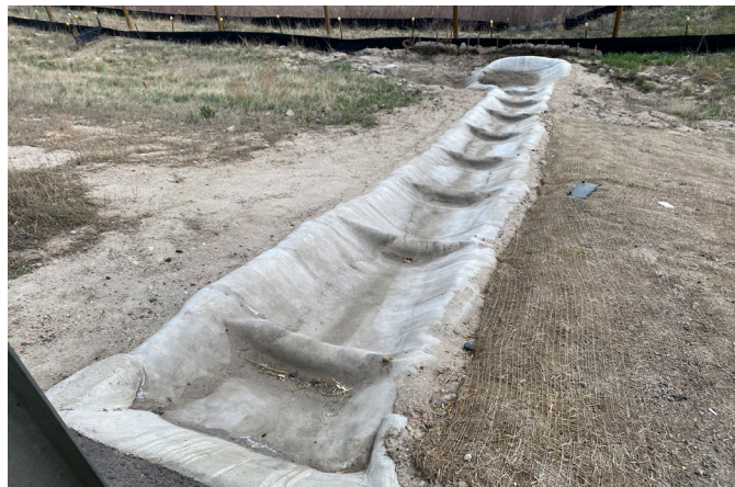
Check Dams & Dissipation Pond Covered in Concrete Canvas®
