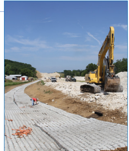
5 Upstream toe of the Flexamat buried in an anchor trench to prevent undercutting.
