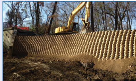
3 Geoweb wall supporting track hoe during infill.
