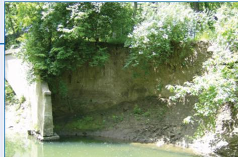
1 Pre construction photo showing the abutment erosion and the loss of the trail.
