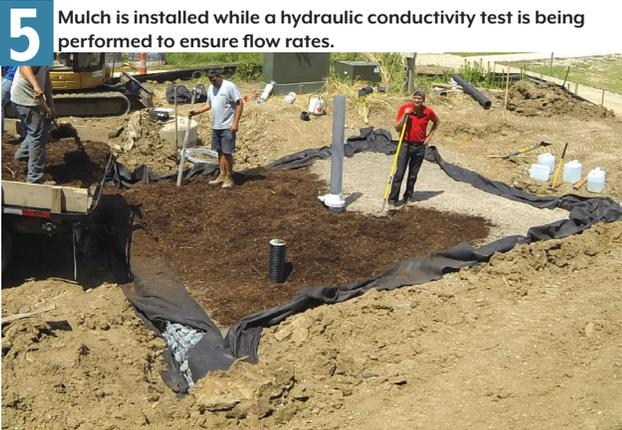
**5** Mulch is installed while a hydraulic conductivity test is being performed to ensure flow rates.
