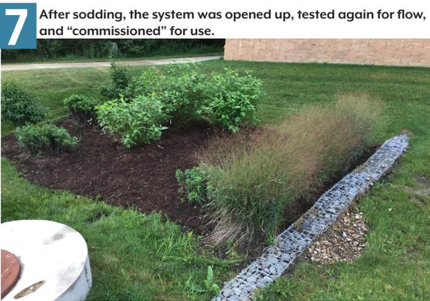
**7** After sodding, the system was opened up, tested again for flow, and "commissioned" for use.
