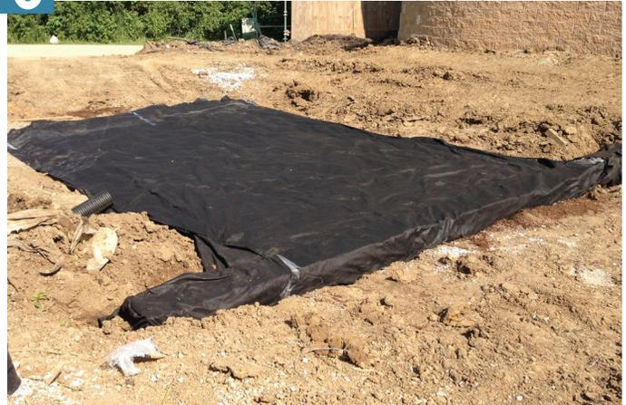
**6** Since ground around Focal Point is not stabilized, the system is completely sealed off to keep sediment from plugging it.
