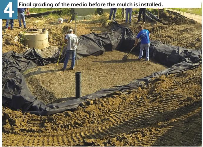
**4** Final grading of the media before the mulch is installed.
