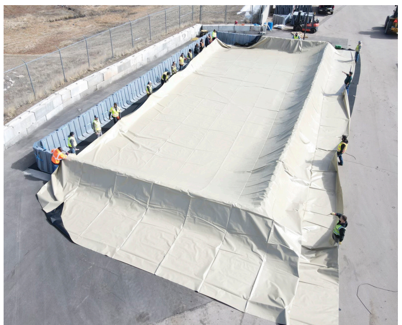
Installing XR-5 liner over the Muscle Wall.
