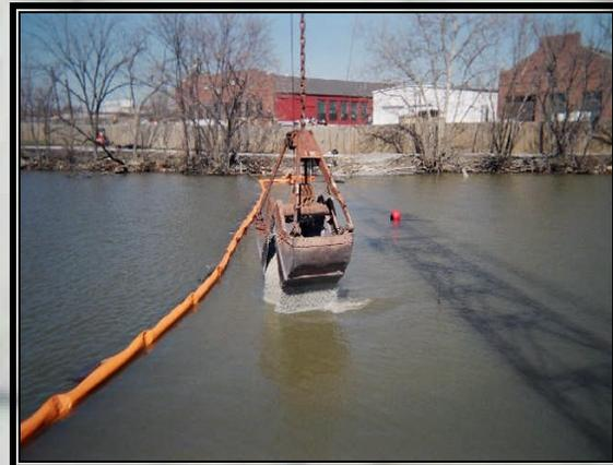
Provided the product is kept dry, AquaBlok® can be handled much like crushed stone aggregate. Conventional methods and equipment can be utilized to apply the material in a broad range of environments and circumstances.
