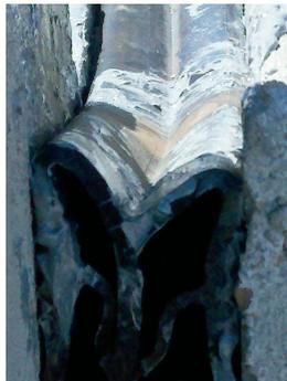
**Step 9 -** Check the ribs for proper adhesive coverage and fill any voids. Excess adhesive above the ribbed area should be removed with a trowel or putty knife.
