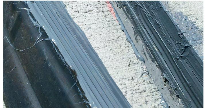
**Step 7 - Apply the adhesive to both vertical sides of the expansion joint and into the ribs of the J or JP Seal.** Apply the adhesive to the sidewall ribs of the profile using a trowel or putty knife as the seal is installed. The ribs must be completely filled with adhesive.
