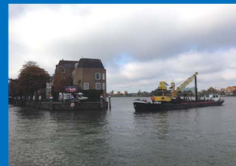
Netherlands 2014 scour protection
