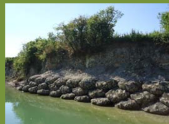
Czech Republic 2013 bank protection
