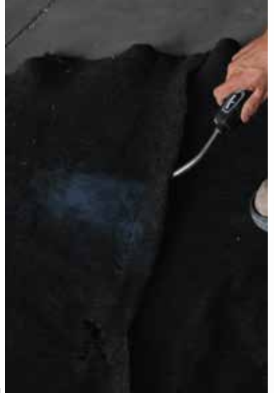
Figure 29: Geotextile being melted together with a torch.
