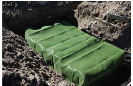
Figure 15 (Above): 12" overlap of Biaxial Mesh on top of underdrain module
