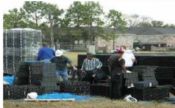
Figure 3: Assembling on site during excavation will increase speed once the excavation is completed
