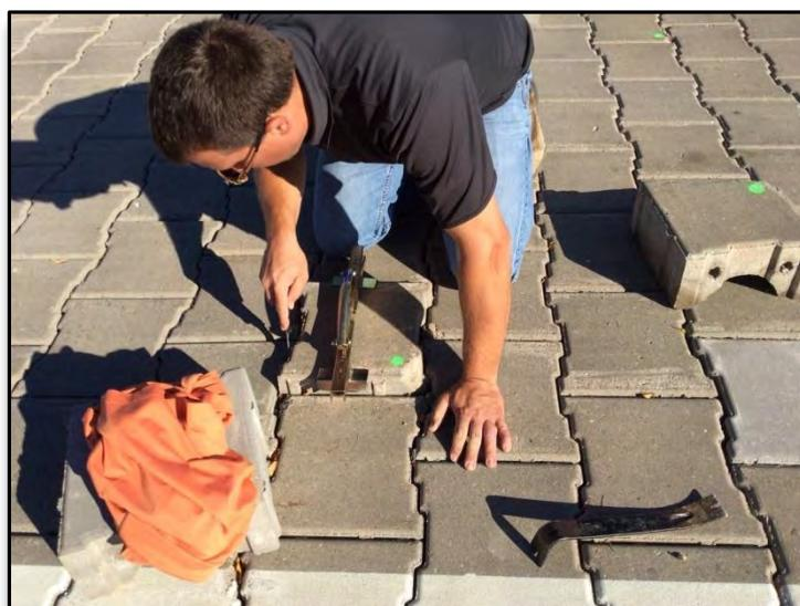
*\*\*The Polyester cables (as shown in Step 1 above) can be cut and removed. It will not affect the performance of the PaveDrain system.*
