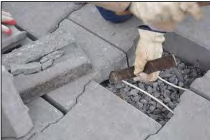
Break out the block using a 3 lbs. hammer, being careful not to damage any of the adjacent blocks. It is best to start in the middle of the block and work your way out. A concrete masonry chisel can help as well.
