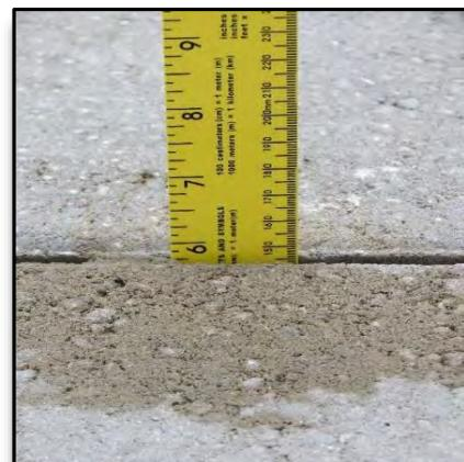
The last resort for maintenance of the PaveDrain System is the removal of the blocks/mats and the subsequent cleaning of the aggregate layer. Once cleaned, then everything is re-installed as a sustainable stormwater solution.
