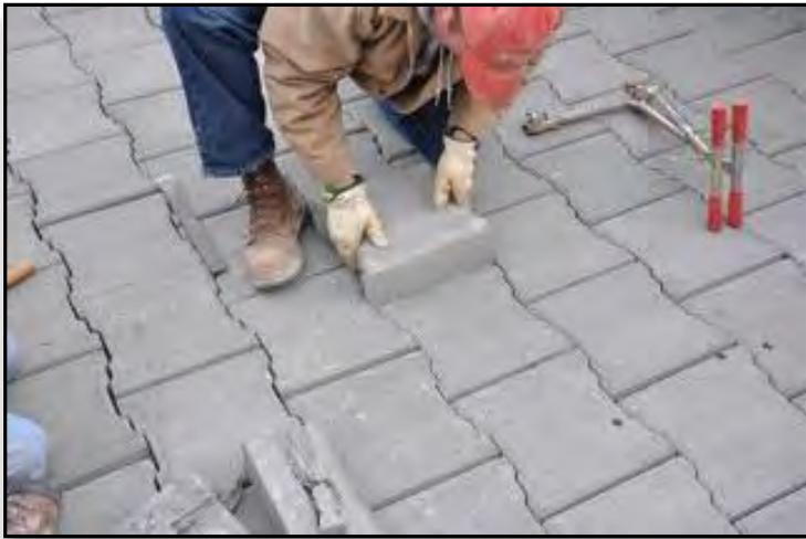
Slide the new block down into place. You may use a rubber mallet to tamp it down securely at the edges, be sure not to damage the new block by using your 3 lbs. hammer!
