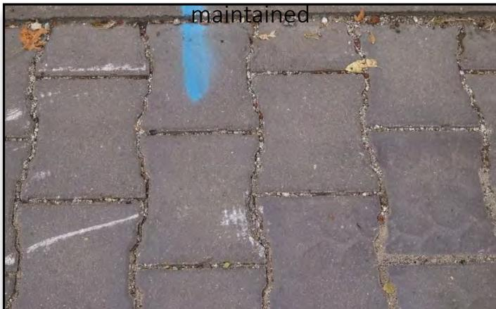
Photo 2 – PaveDrain following maintenance
