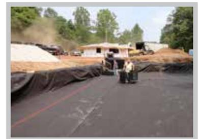
Fig. 7 Use a string line and marking paint to square the system footprint.
