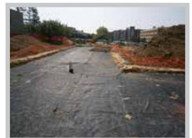
Fig. 25 Overlap Geogrid 18" or as required by plans.
