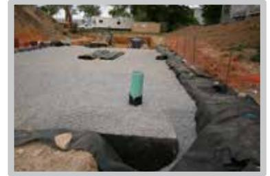
Fig. 24 Use an LGP dozer to push backfill over R-Tank® units.
