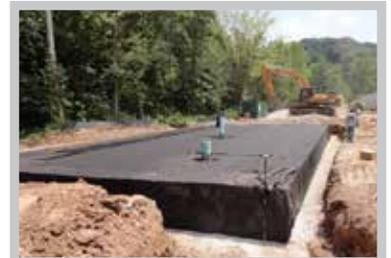
Fig. 21 Finished envelope should lay flat against R-Tank®.
