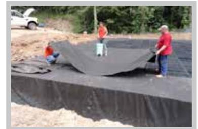
Fig. 20 Encapsulate R-Tanks® with geotextile.
