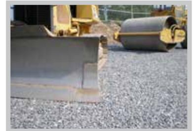
Fig. 4 Base must be smooth to ensure units fit together without gaps.
