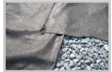
Fig. 6 Reduced overlaps don't create significant savings and can create delays.
