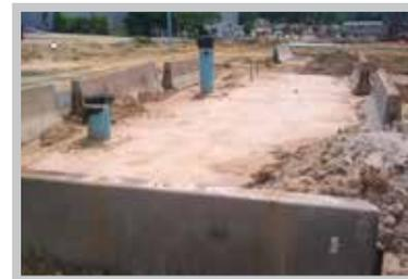
Fig. 28 Secured R-Tank® installation using Jersey Barriers.
