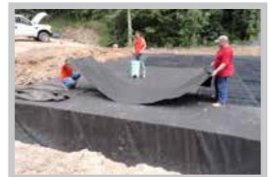
Fig. 20 Encapsulate R-Tanks® with geotextile.
