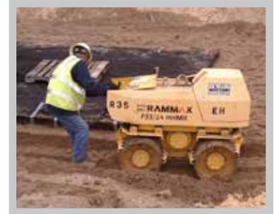
Fig. 23 Vibratory compaction of side backfill is ALWAYS REQUIRED, regardless of what backfill material is used.
