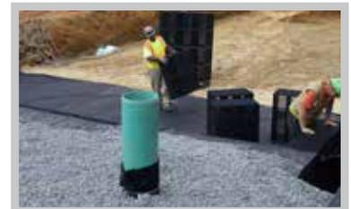
Fig. 11 Installed Inspection Port
