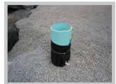
Fig. 17 Install port into R-Tank®.
