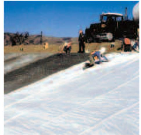
Hydrotex Linings, Mats, and Armor Units are filled in place by pumping fine aggregate concrete into fabric forms. The results are reduced material and equipment costs, faster installation, and dependable erosion and scour prevention.
