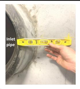
6) Make a horizontal mark from center of pipe, crossing bracket marks from previous step.
