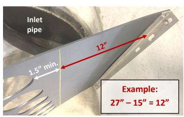
13) If determined necessary in Step 12, make a <u>straight cut</u> along the cut line. Remove scrap from bracket and retain screws.
