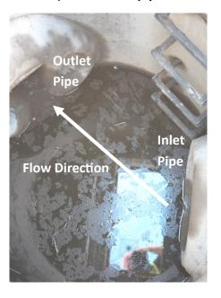
4) Inspect bracket locations - 9" ± from inside of pipe - and remove/avoid any obstructions.
