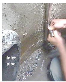
9) Install one anchor bolt per pair of slots. See additional anchor bolt instructions in hardware bag. Repeat Steps 6 through 9 to attach the other wall bracket.
