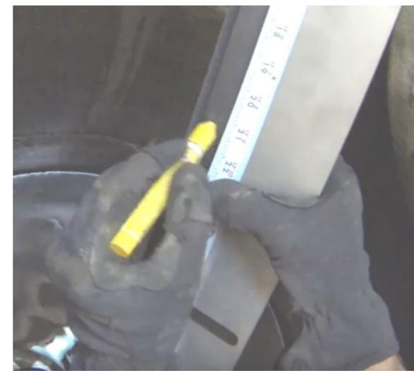
7) Measure and mark the center of the wall bracket on the back (pipe side) edge.
