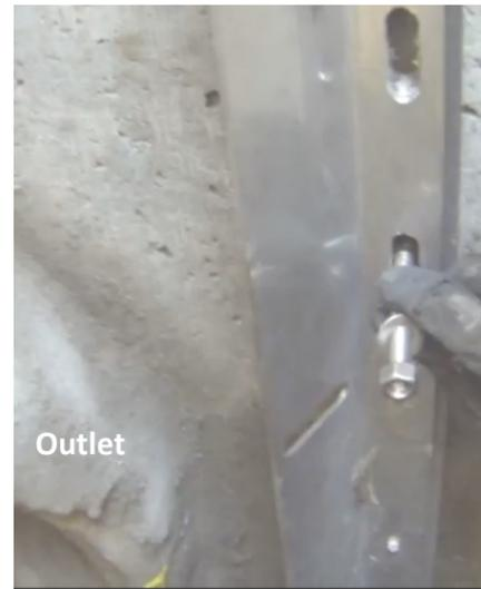
10) Working from the bottom up and leaving nuts and bolts loose, attach arches to wall brackets. Go to next step prior to attaching top arch.
