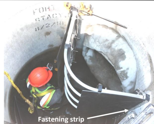
14) Attach both side sheets at wall using (2) fastening strips and provided screws. Use hand clamps for assistance. Apply pressure and adjust your drill's torque setting to prevent stripping.
