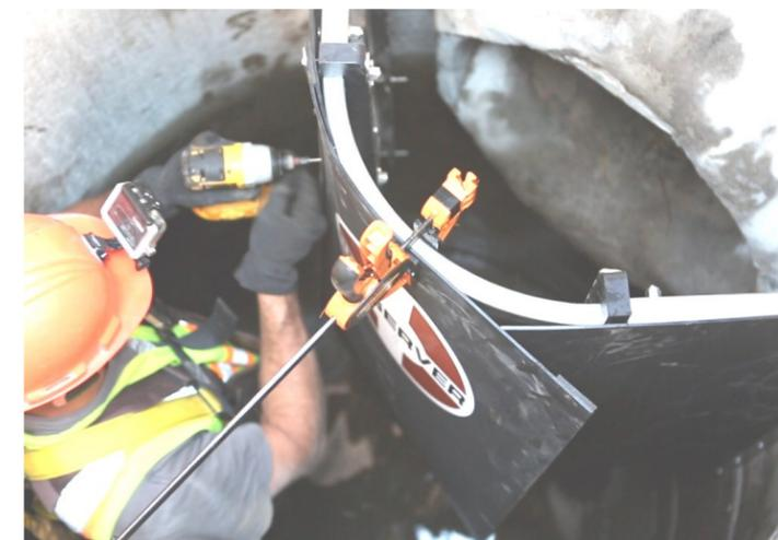
15) Clamp center sheet to center of skimmer structure, overlapping side sheets as shown above. Attach center sheet to vertical supports using (2) remaining fastening strips and provided screws.
