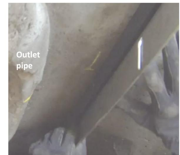
8) Align wall bracket with marks made in Steps 5, 6 and 7. Use level to ensure bracket is vertical prior to next step.
