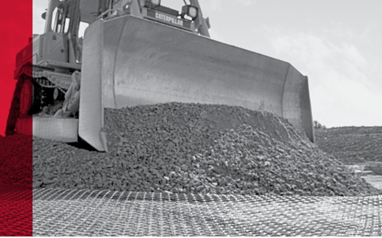
IMAGE 8: Dumping aggregate fill on top of Tensor® Geogrid over competent subgrade.
