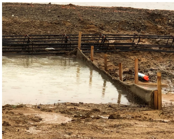
Shown Left to Right: Straw wattle deformation as degradation occurs, WattleFence in action under sediment-laden flows, WattleFence continued performance after multiple flow event.
